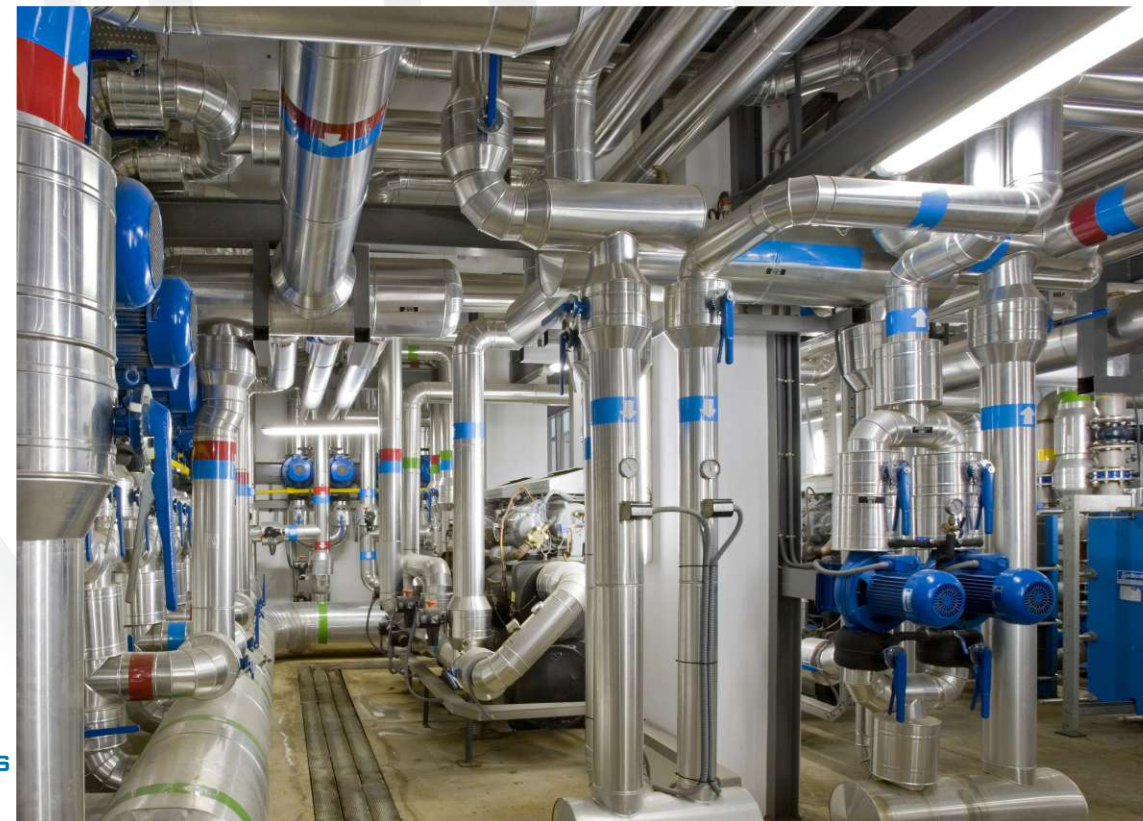
ANDALUSSIAN PARLIAMENT (SEVILLE) ENGINE ROOM - HVAC SYSTEM APPLYING GEOTHERMAL TECHNOLOGY
